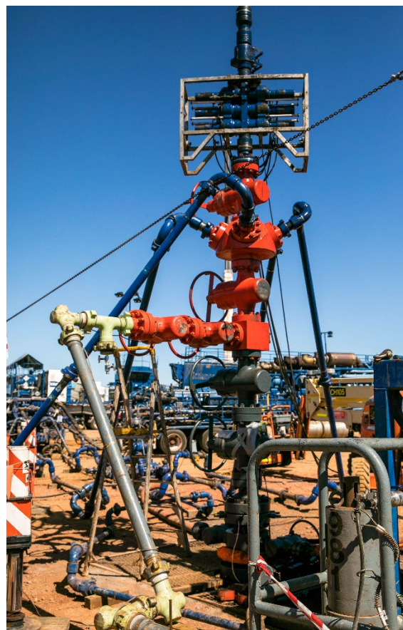
Carpentaria-2H high-pressure hydraulic stimulation wellhead
