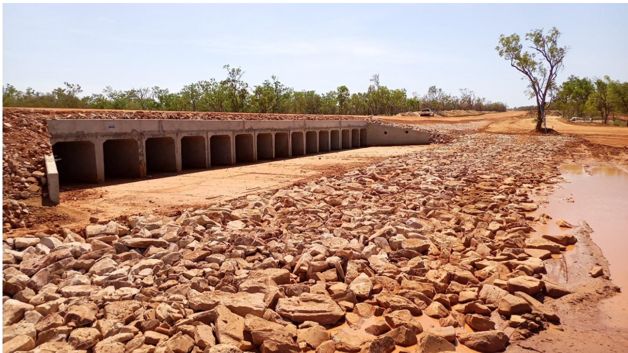
Figure 3: Thunderbird mine access road – culvert installation
