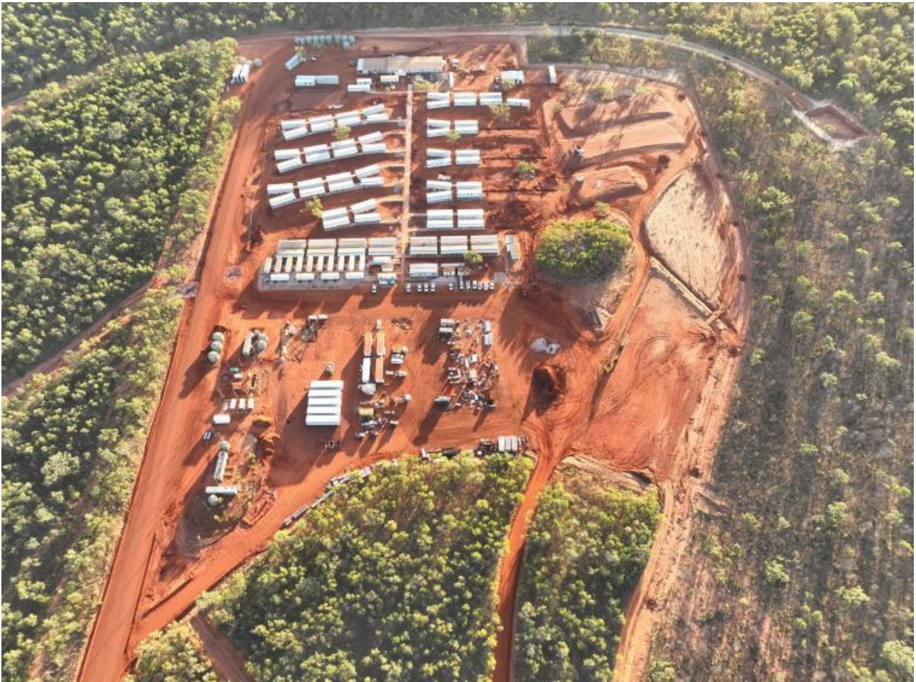
Figure 4: Thunderbird village accommodation – under construction
