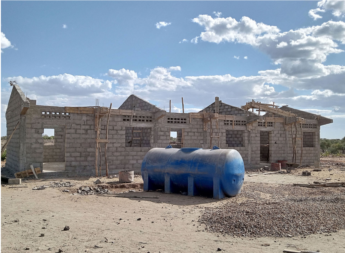
Figure 3 – Progress of School Construction in August 2022
