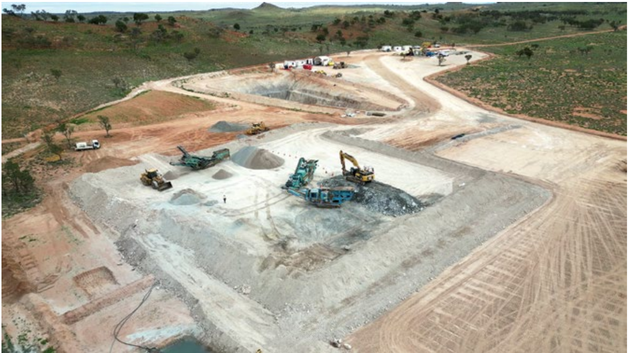
Figure 8 – Multi-stage crushing plant processing ore stockpile in preparation for milling.
