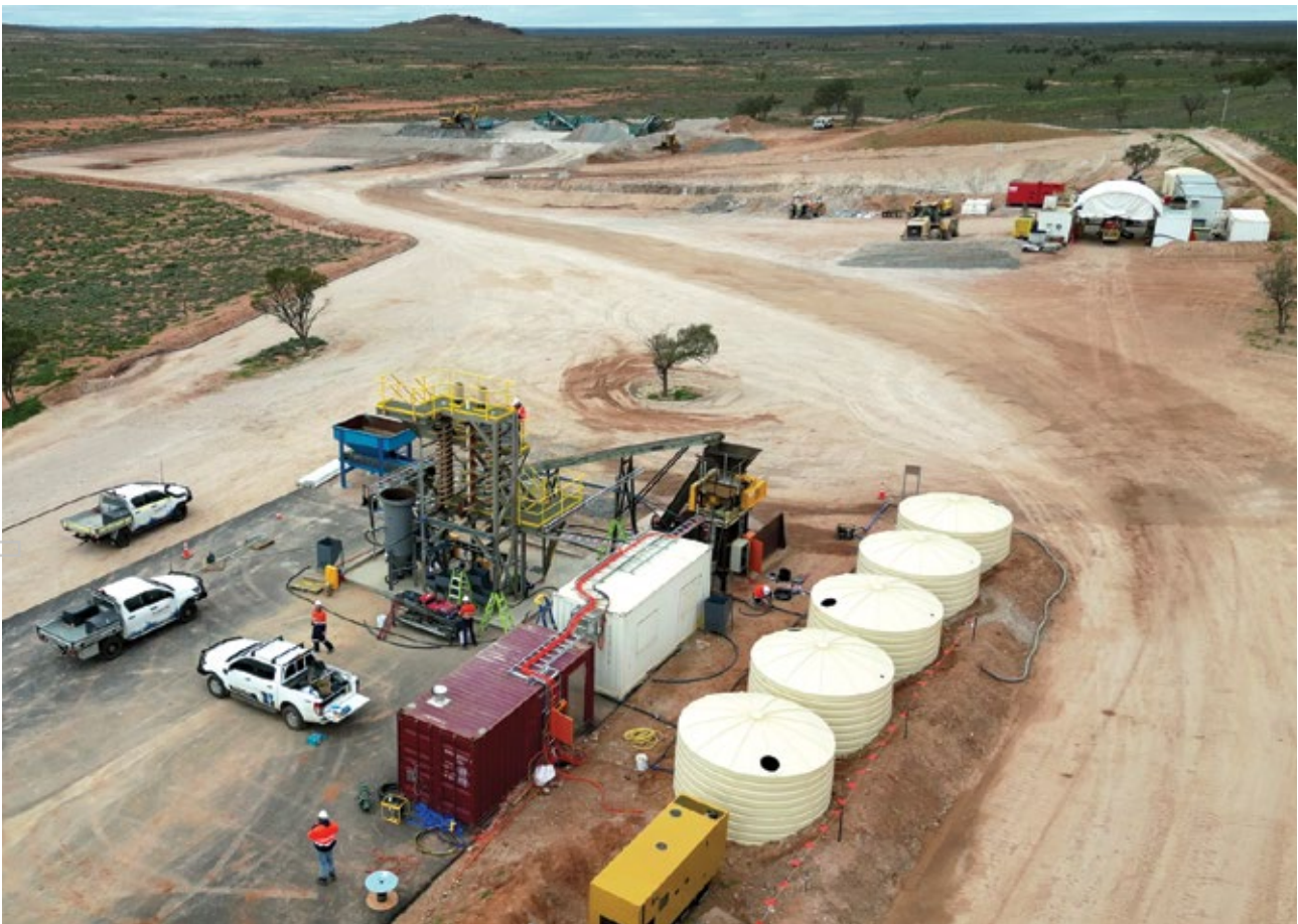
Figure 7 – Pyrite Hill site concentrator including gravity spirals.
