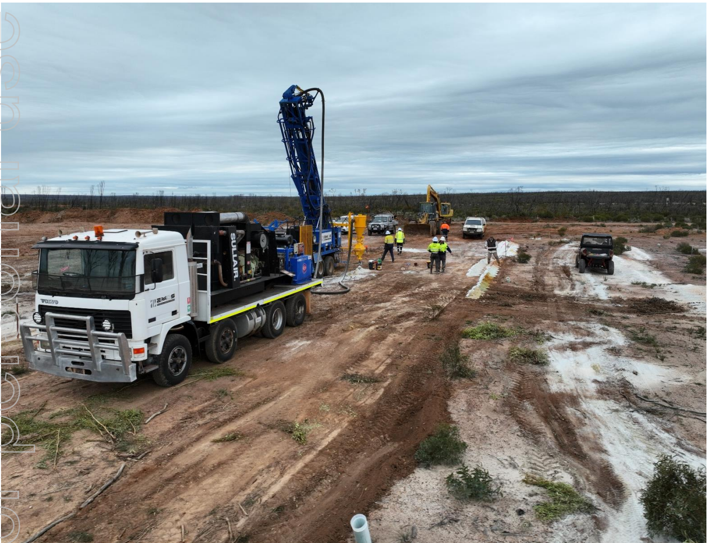
Figure 2: Infill RC Drilling at Kat Gap
