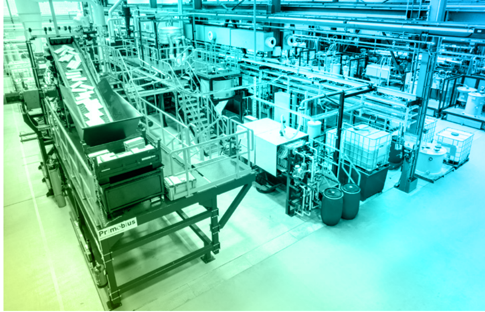
Shredder and beneficiation processing EV cells
