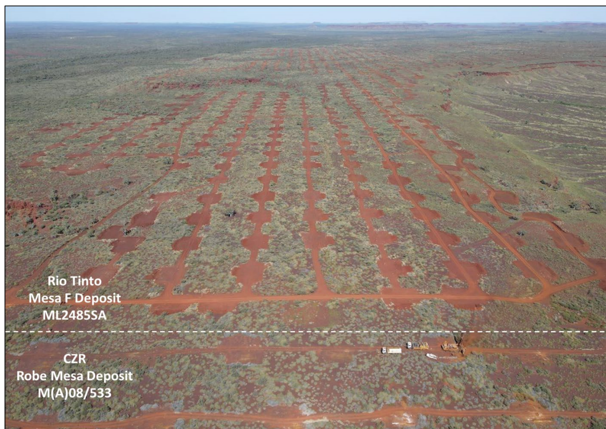
Figure 7. CZR's Robe Mesa deposit in the foreground with RC drill rig, with Rio Tinto drill lines and pads cleared to the CZR tenement boundary (19 July 2022)
