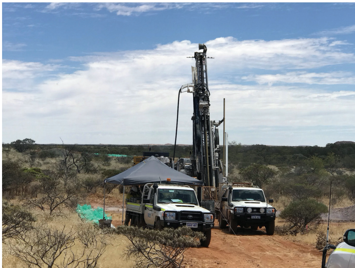
Figure 19: RC drill rig at Four Corners prospect
