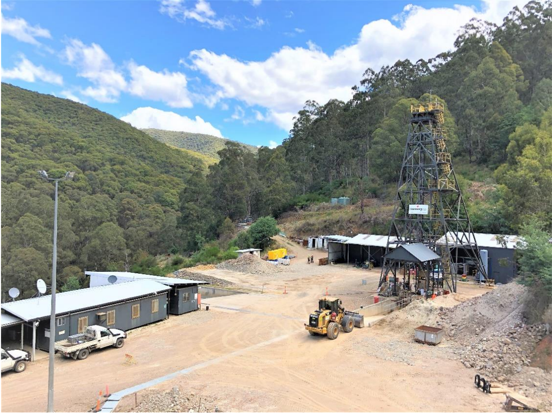
Figure 2: Morning Star mine site with headframe and winder on the right and offices to the left
