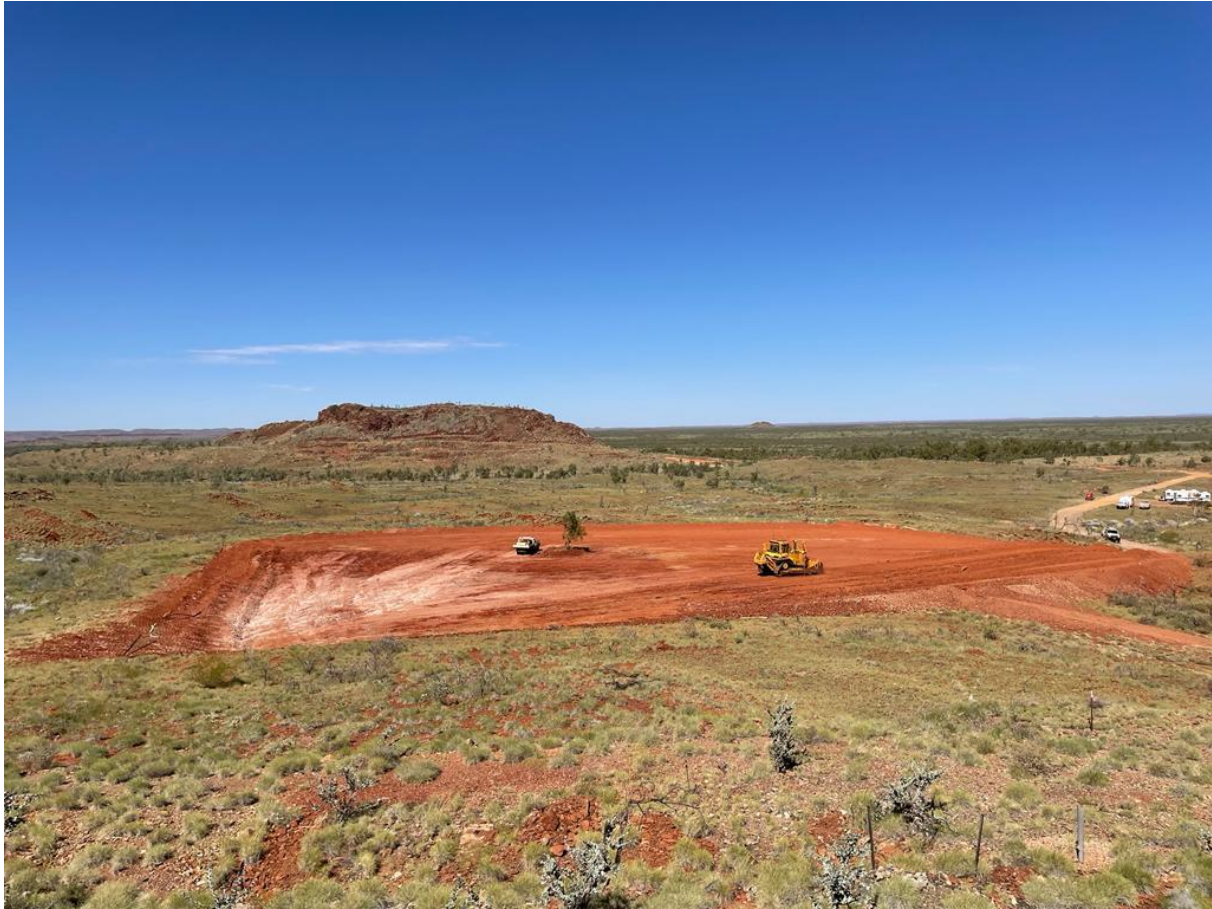
Figure 13. Exploration camp construction underway with levelling and compaction of 70m x 70m area in preparation for dome-sheltered core yard, accommodation, ablution block, workshop and offices. The prominent hill in the background is the part of the Main Hill prospect. View looking south.
