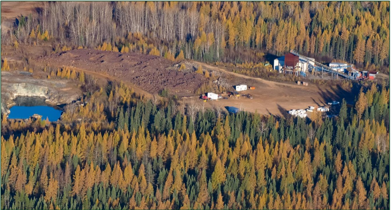
Image 2: Pickle Crow processing plant
