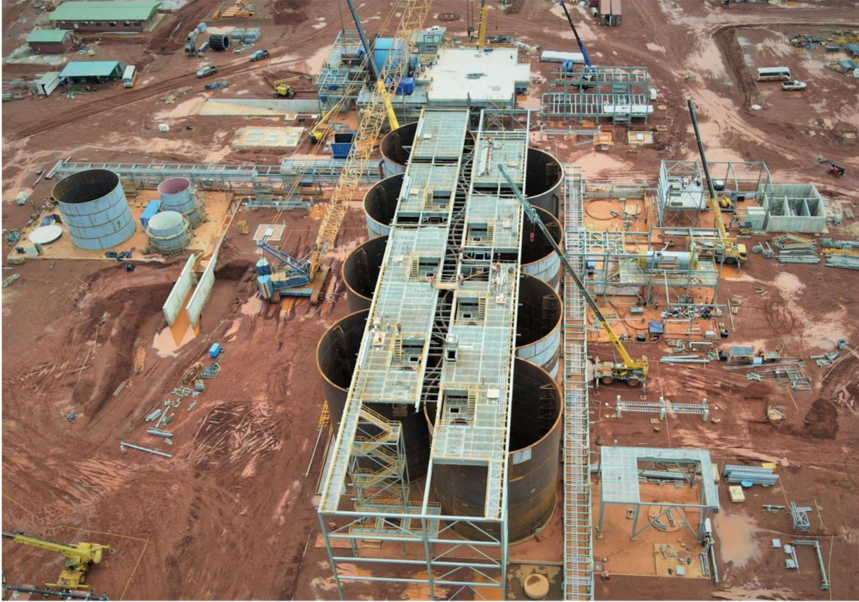
Figure 4 CIL tanks installed
