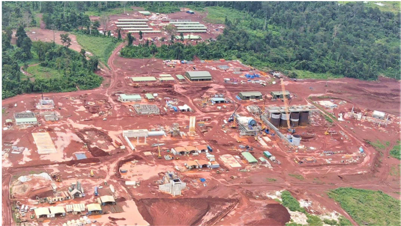
Figure 2 Overview of the Abujar Gold Mine processing plant and mine camp as of early September 2022
