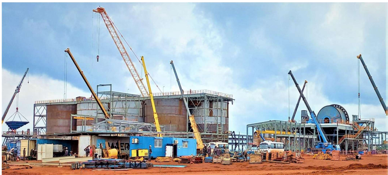
Figure 3 SAG Mill installation as of early September
