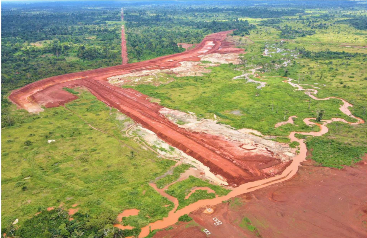
Figure 7 Water dam and water diversion channel
