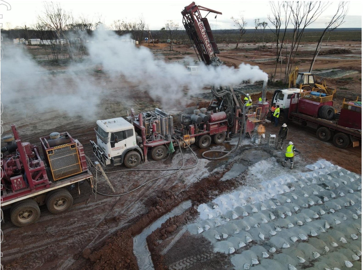
Figure 4: RC Drilling at Kat Gap
