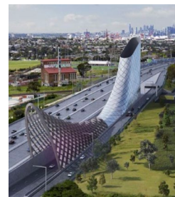
Westgate Tunnel Switchboards – Trivantage Manufacturing Over $10m
