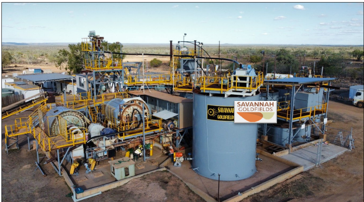
Georgetown Gold Processing Plant
