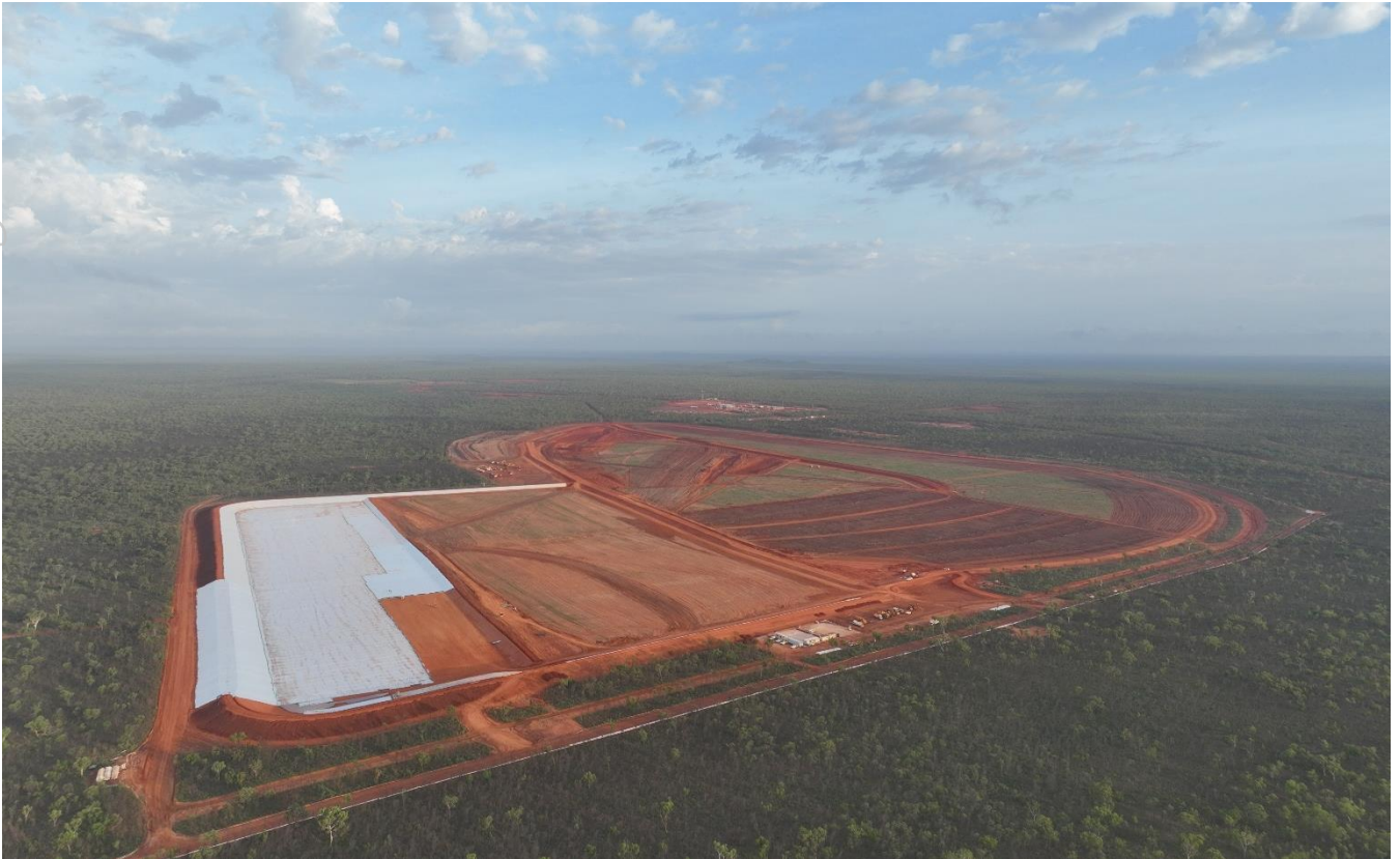
Image 3: Lining of the Stormwater Storage Pond underway
