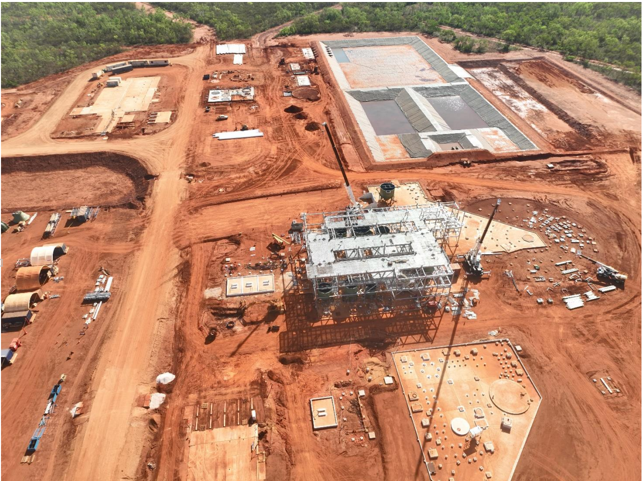
Image 1 & 2: Thunderbird Plant Site Progress – Plant steel erection and process tank installation
