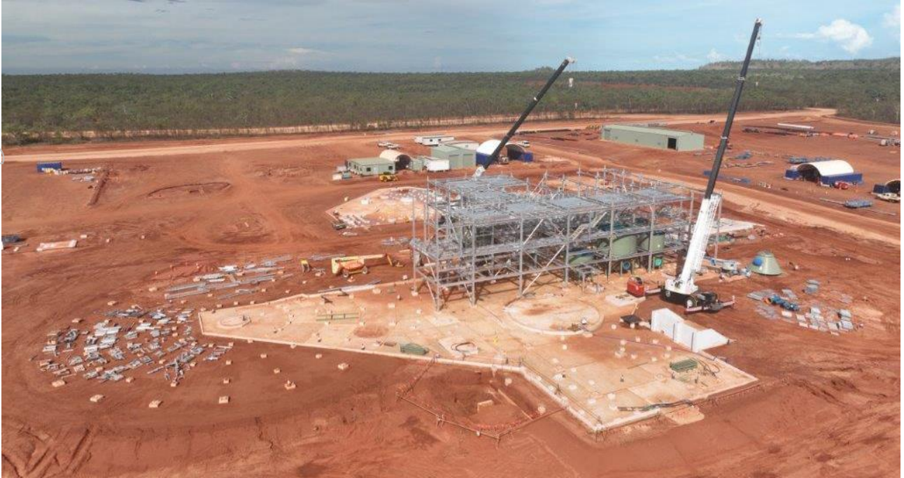
Image 1 & 2: Thunderbird Plant Site Progress – Plant steel erection and process tank installation
