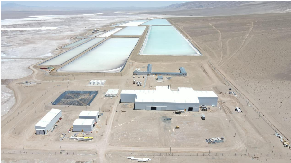
Figure 3. Rincon Lithium Project – 2,000tpa Operations Site
