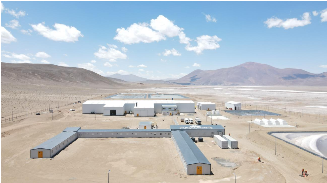
Figure 9. Rincon Lithium Project – 2,000tpa Operations Site
