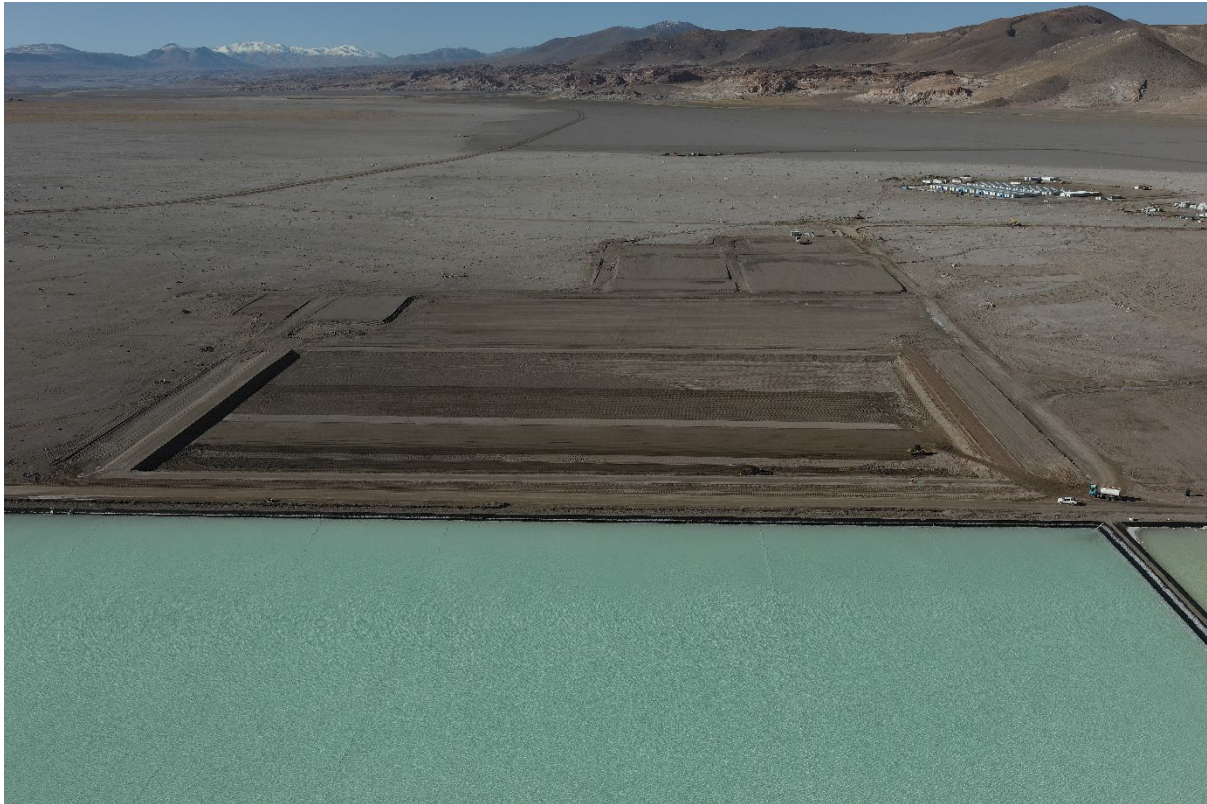
Figure 4: Sal de Vida: Earthworks platform for process plant
