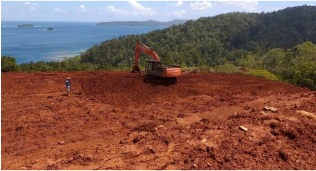
Figure 38 Pit Clearing and Access
