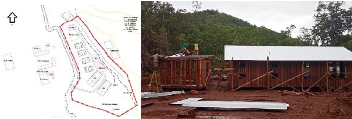
Figure 34 Initial 50 Person Camp Facility
