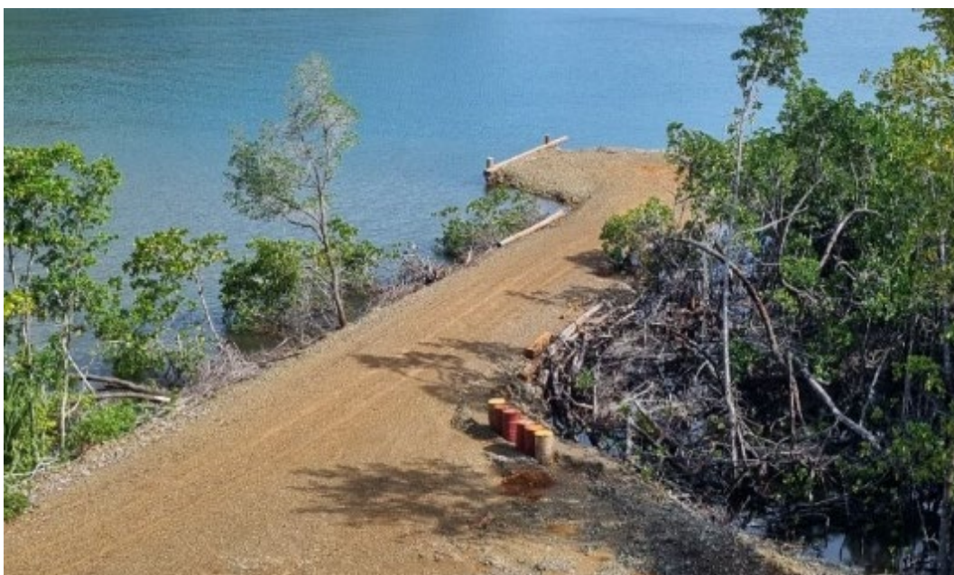
Figure 40 Equipment Landing Wharf
