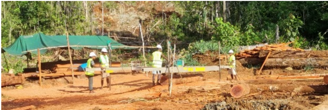
Figure 39 Local Timber Milling On Site
