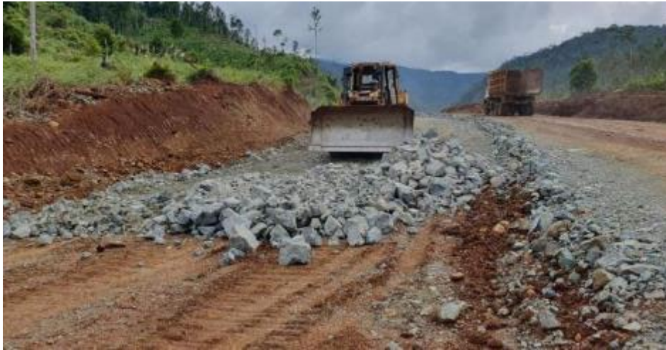
Figure 37. Example – Ni Ore Access & Haul Road Development
