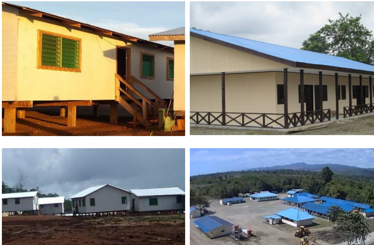
Figure 35 Local and Prefabricated Camp Buildings
