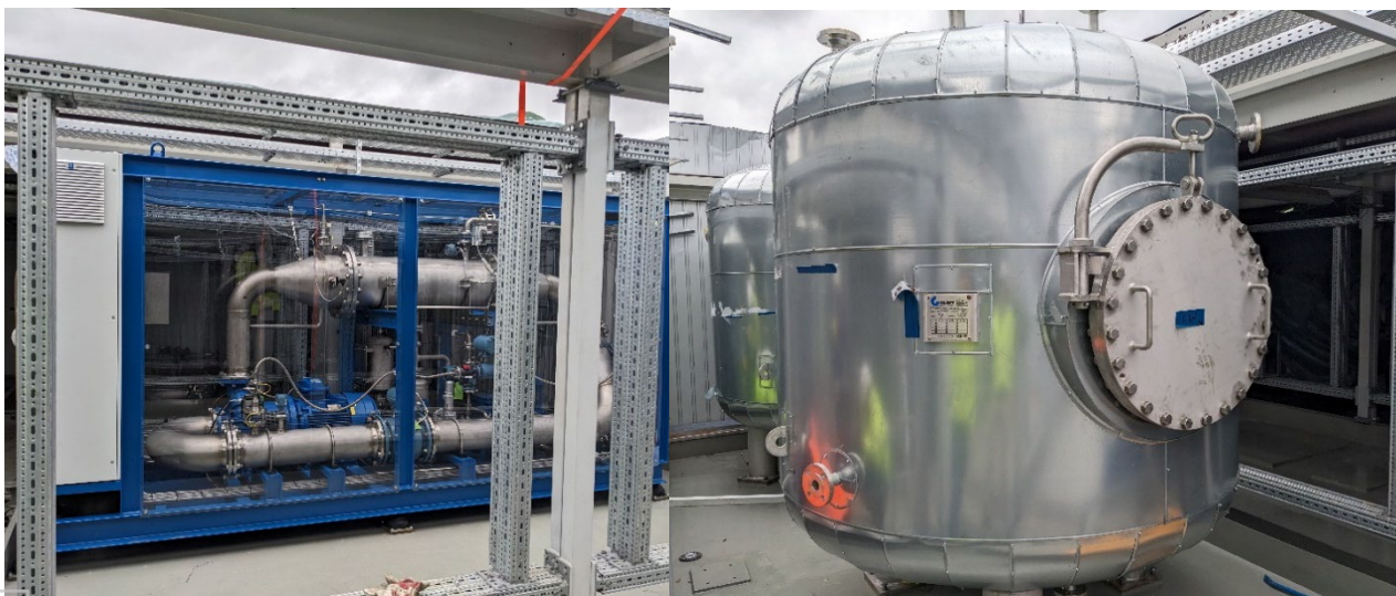
Figure 20: In-house designed lithium extraction Demo Plant, currently under construction.
