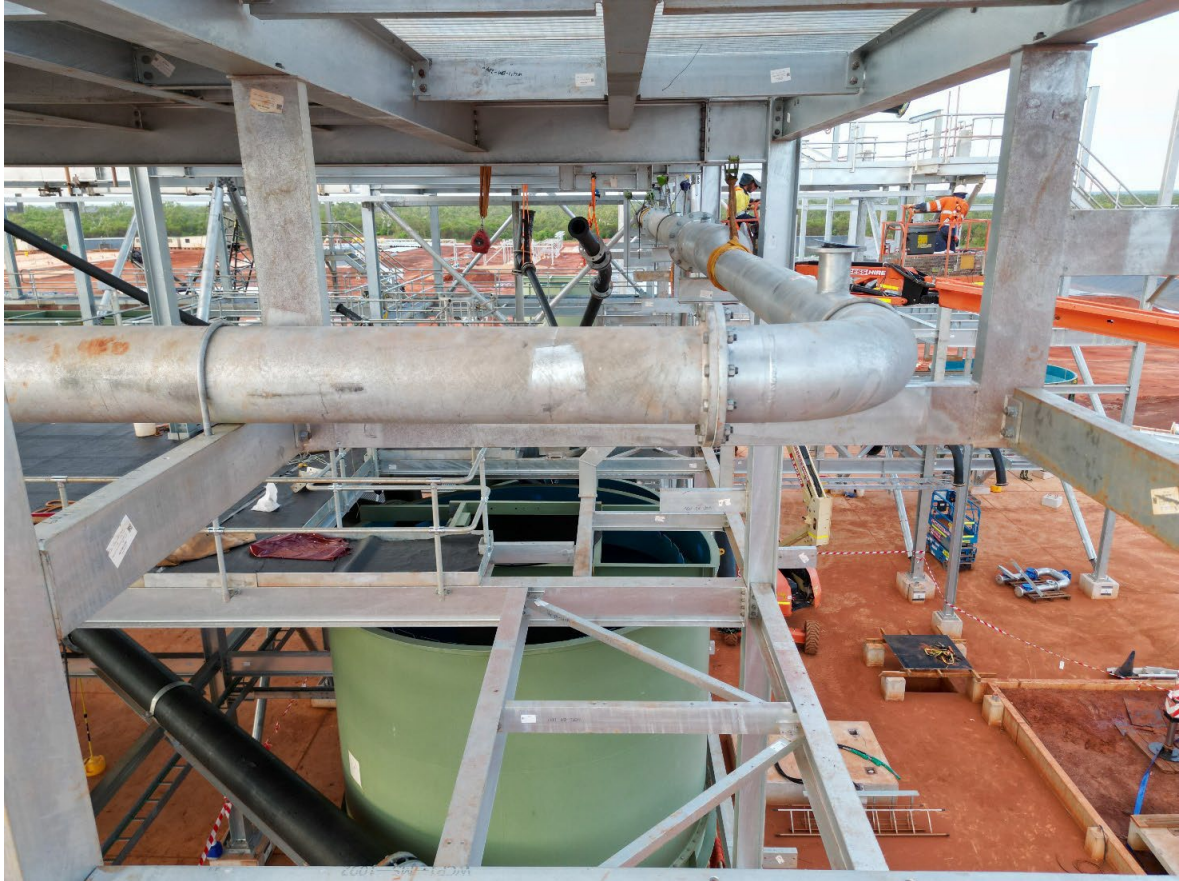
Image 4: Wet Concentrate Plant steel piping installation
