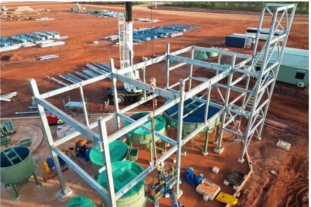
Image 3: Concentrate Upgrade Plant - steel installation
