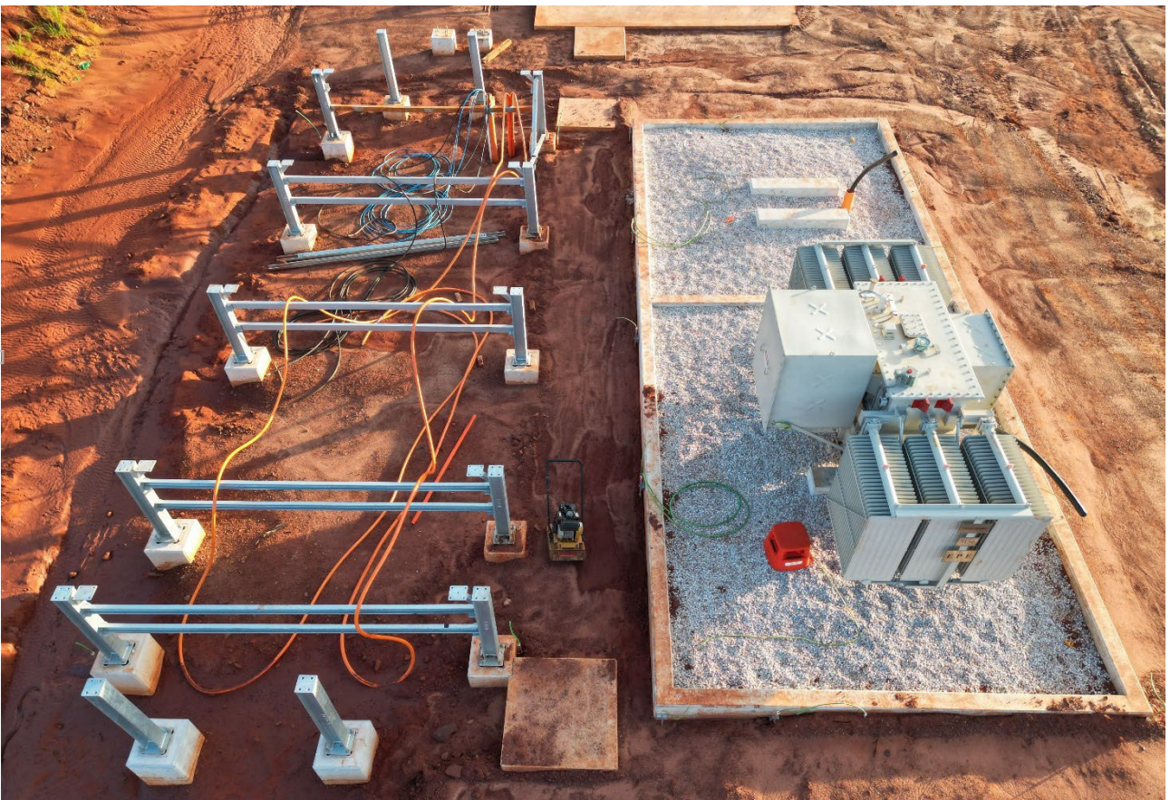
Image 7: Process Water Area sub-station – electrical works
