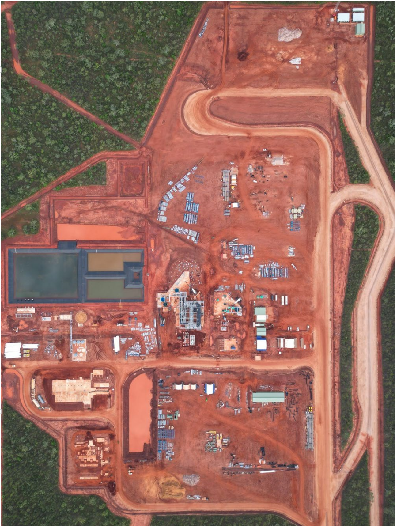
Image 1: Thunderbird Plant Site – aerial view (February 2023)
