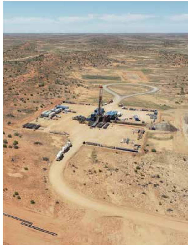
Drilling of CCS injection wells
