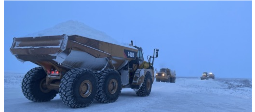
Ice road construction
