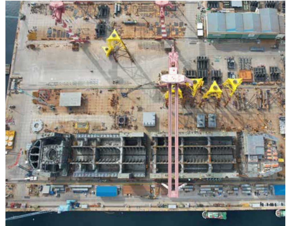
Barossa FPSO construction
