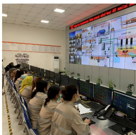
Control room at Angel Nickel
