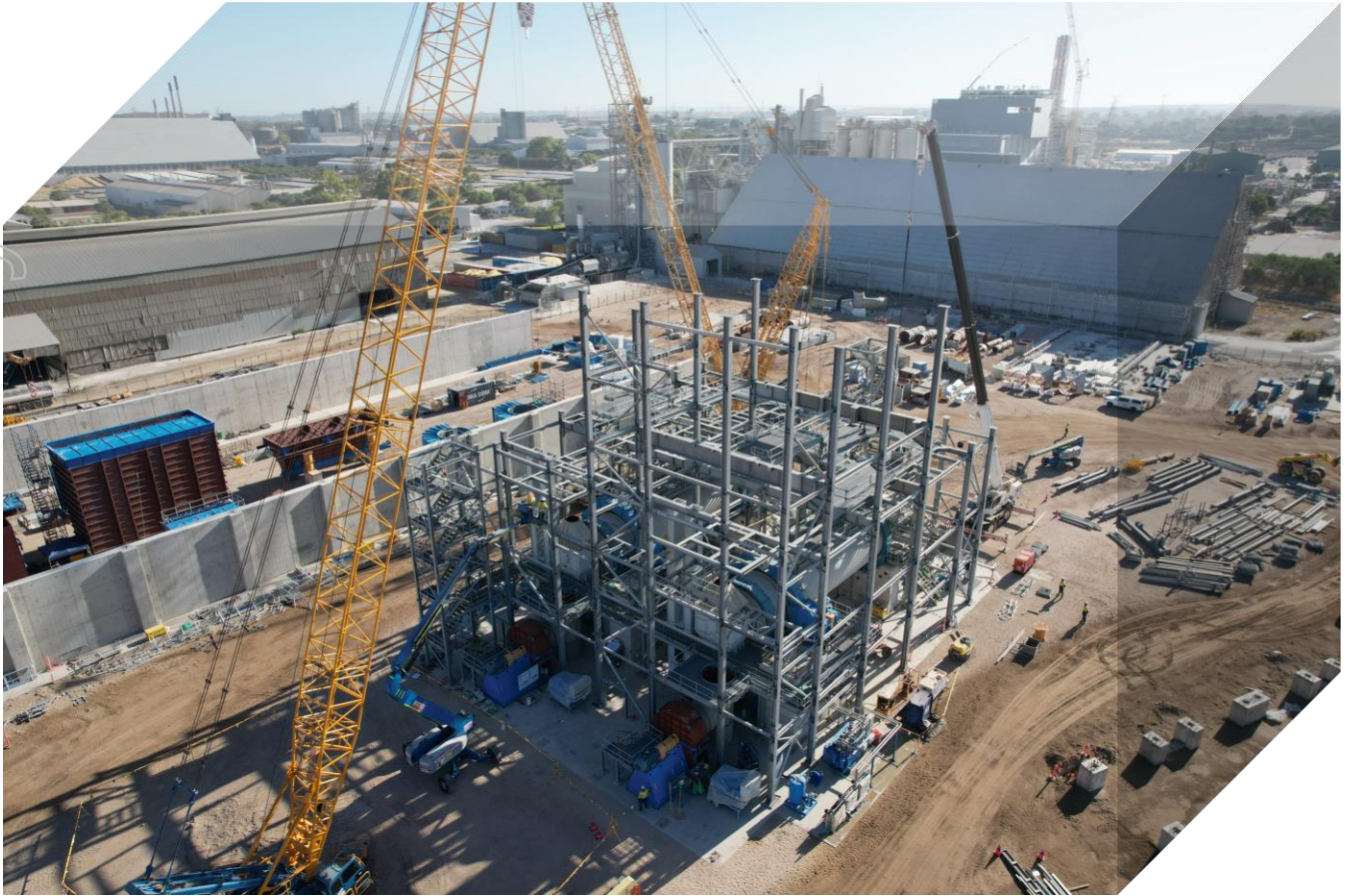
Image: Cockburn Cement Kwinana Upgrade Project (SIMPEC)
