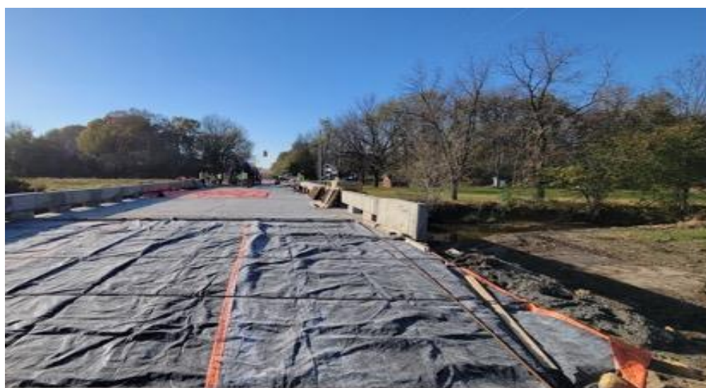
Figure 5. EdenCrete® bridge trial in Clinton County, Iowa
