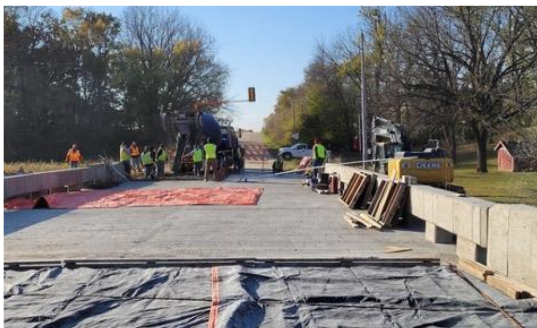
Figure 4. EdenCrete® bridge trial in Clinton County, Iowa
