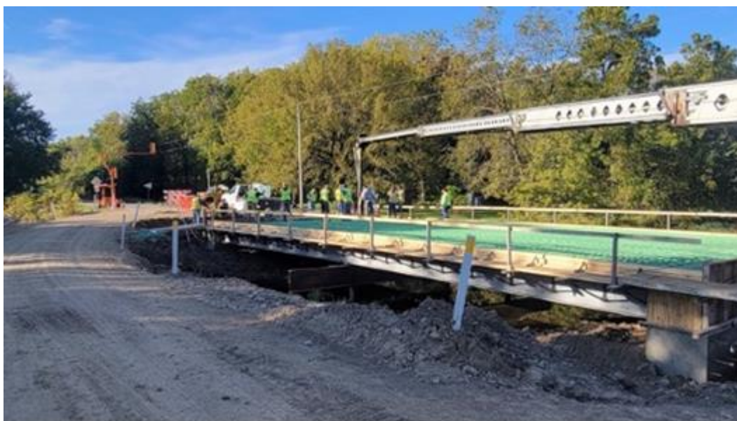
Figure 3. EdenCrete® bridge trial in Clinton County, Iowa
