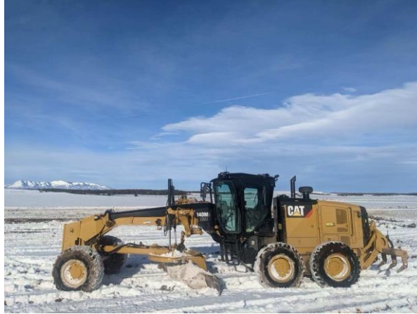
Figure 5: Jesse-2 well pad construction begins in Utah
