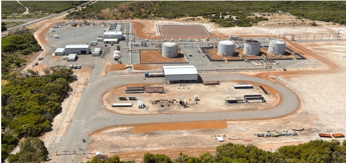
Figure 1: Arrowsmith Stabilisation Plant (ASP)
