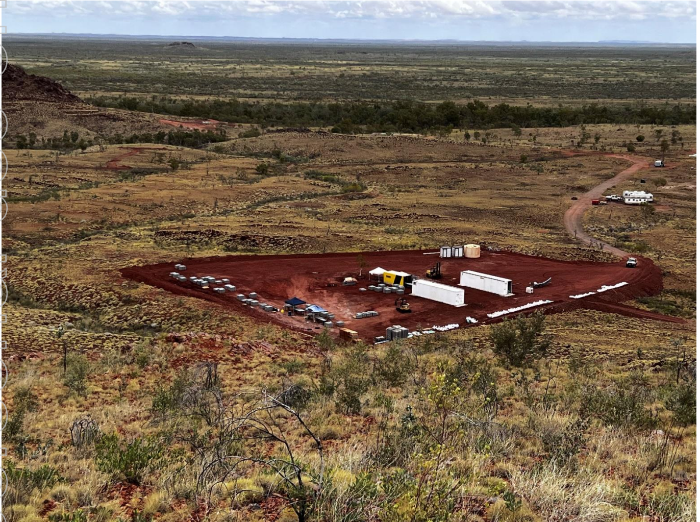
Figure 16 - Exploration camp construction underway with levelling and compaction of 70m x 70m area in preparation for dome-sheltered core yard, accommodation, ablution block, workshop and offices. The prominent hill in the background is the western part of the Main Hill deposit. View looking southwest.
