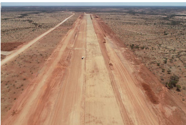
Figure 2. Mine Site Airstrip: nearing completion and first operations.
