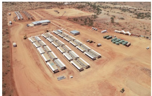
Figure 3. Kurrbili Accommodation Village: Phase 1 and 2 taking shape.
