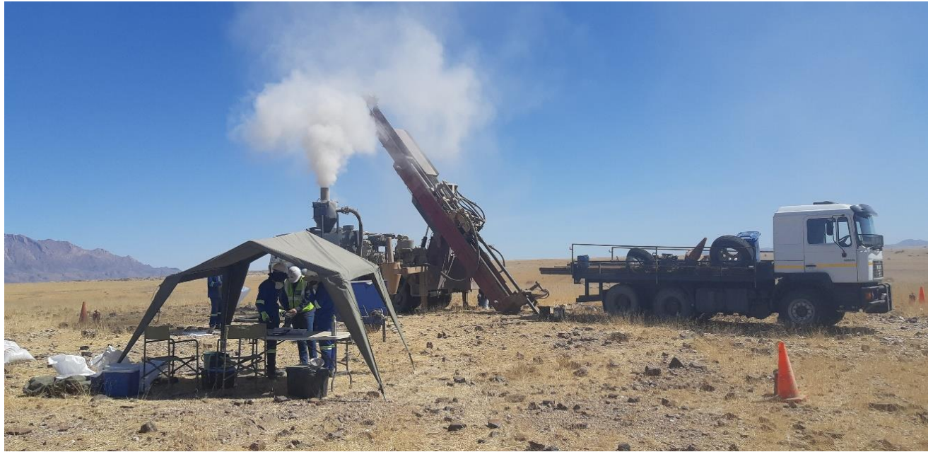
Figure 7: RC drill rig in operation at Area 1 within EPL 8535
