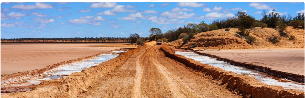
FIGURE 2: CAUSEWAY ACROSS LAKE SURFACE TO FACILITATE DRILLING CAMPAIGN
