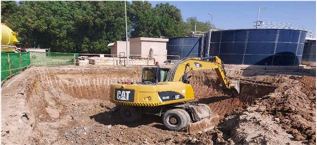
Figure 5: Tank excavation works at the Haya Water site
