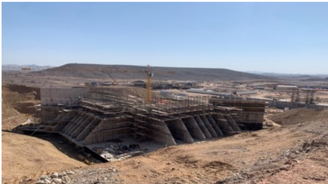
Figure 1: Retention wall and primary crusher
