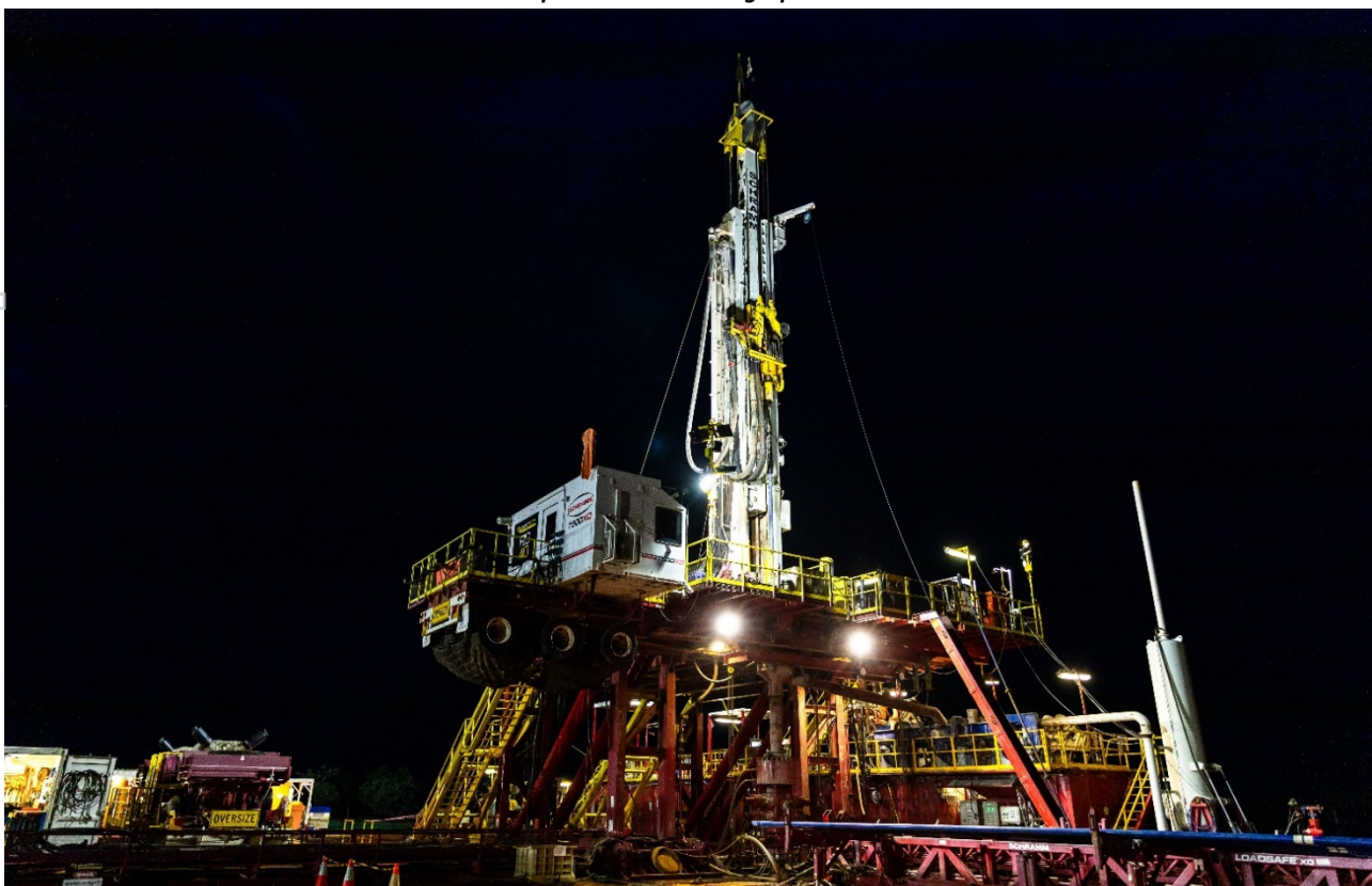
Carpentaria-2H Drilling Operations
