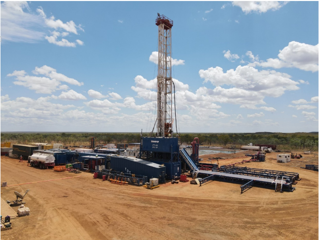
Carpentaria-3H Drilling Operations
