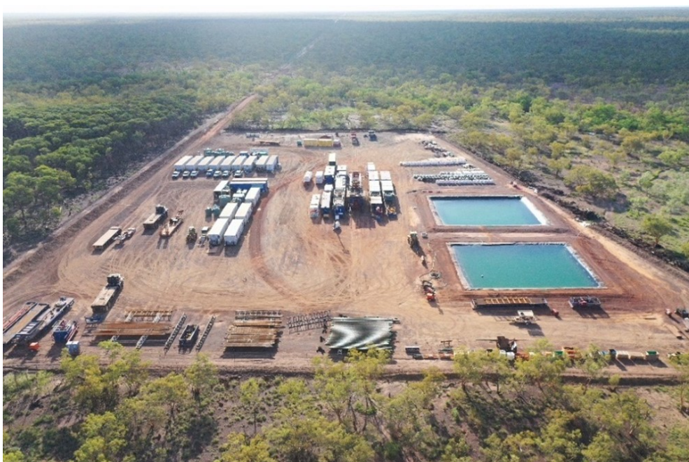
Carpentaria-4V Drilling Operations
