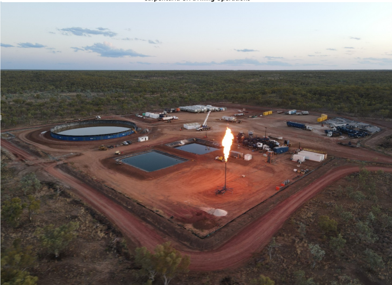
Carpentaria-2H Extended Production Test Flare
