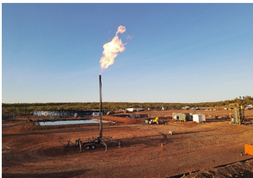
Carpentaria-2H Extended Production Test Flare
