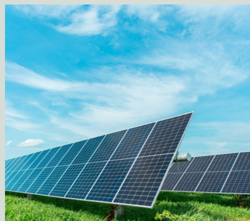
Balama solar and battery project
