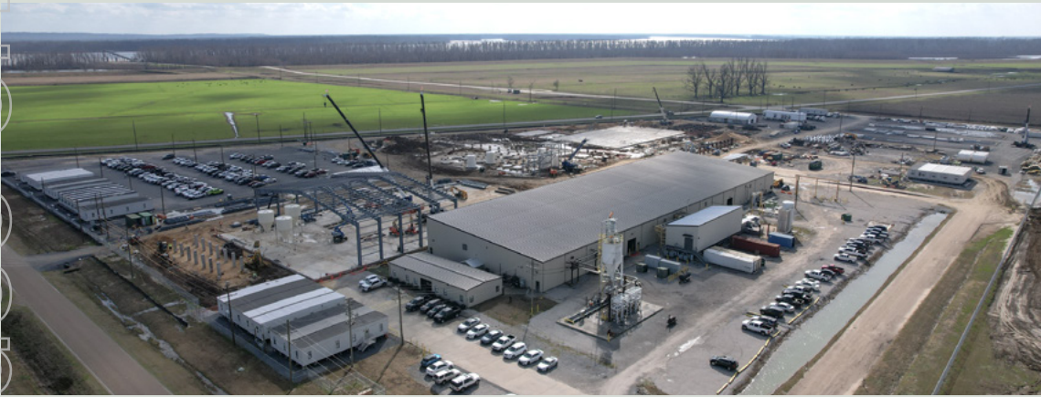
◀ Vidalia AAM facility
