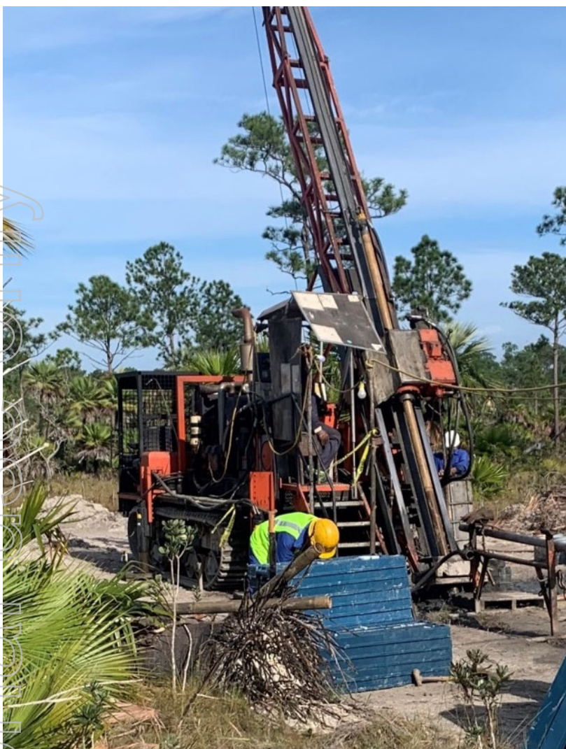
Drilling at La Demajagua
