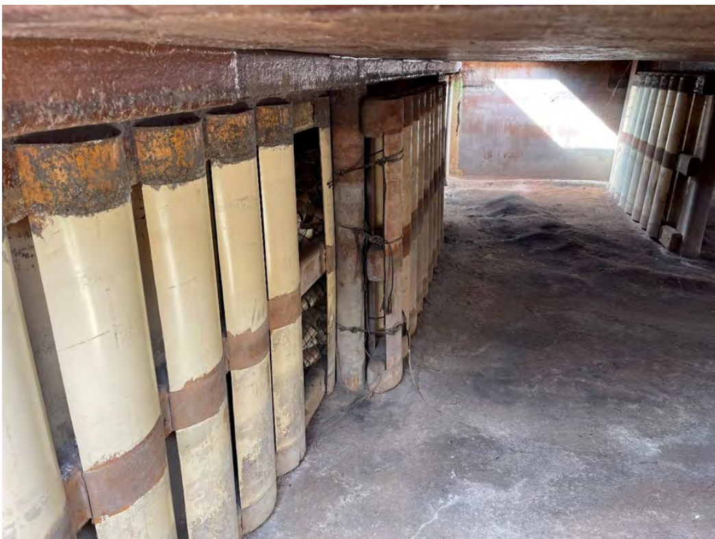
Image 1 / SX Mixer Settler cleanout lower level
