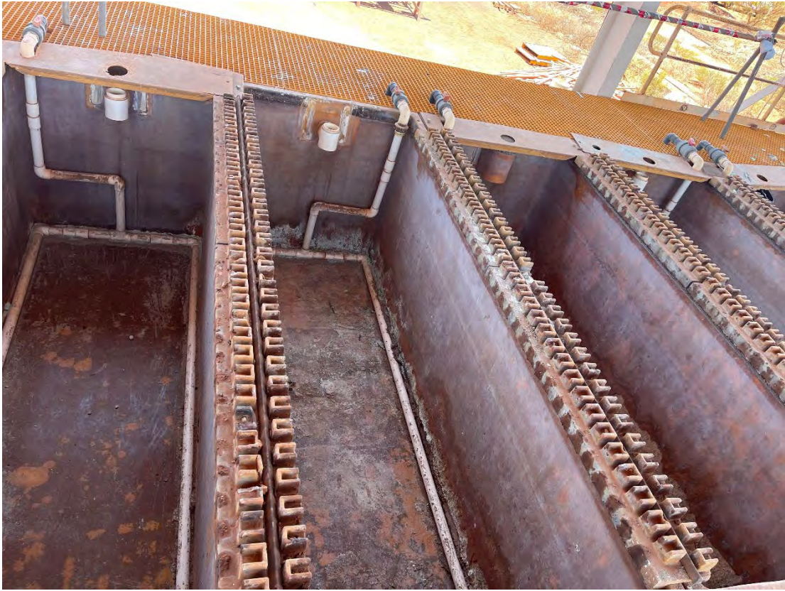
Image 4 / Cleaned EW Cells ready for condition inspection
