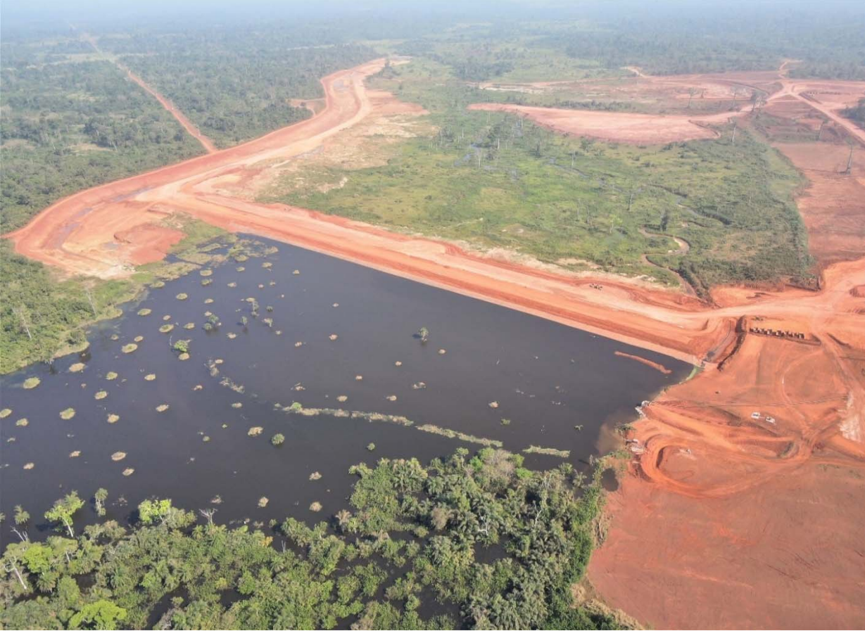
Figure 7: Water storage dam and diversion channel
