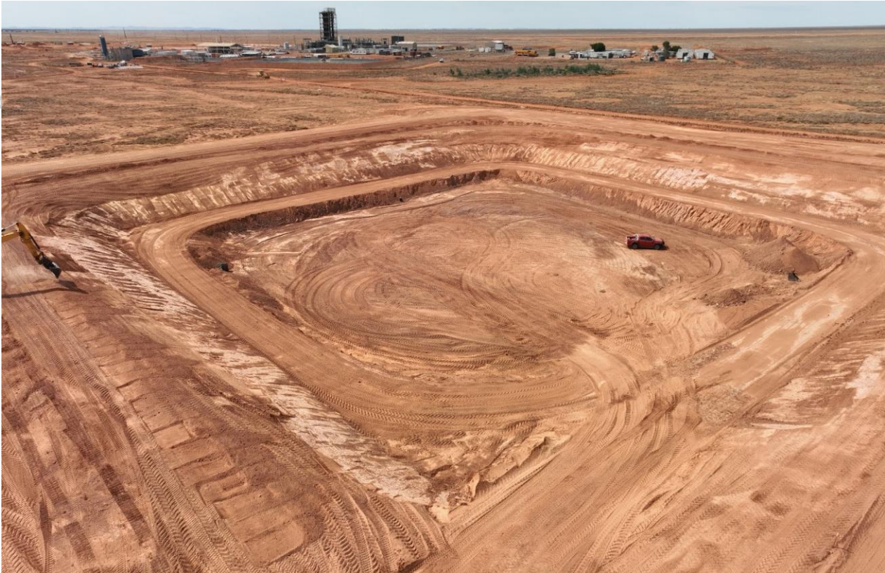
Image 3: 60,000 cubic metres excavation earthworks for the 25,000 ton gypsum pond now complete.
