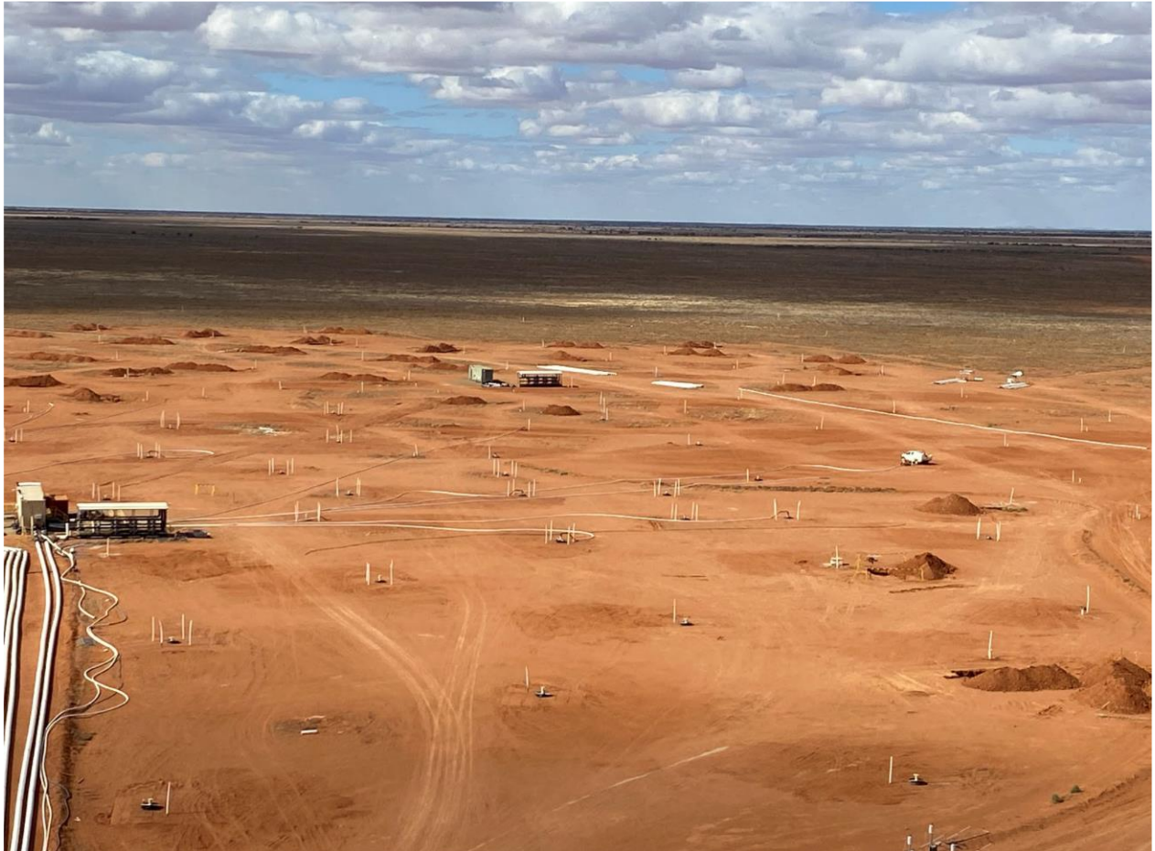
Image 2: Construction of the three start-up wellfields is now ahead of schedule.
