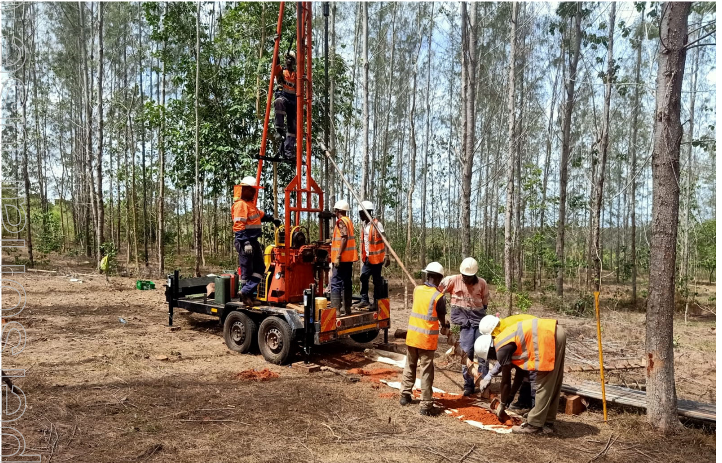
Figure: Auger drill rig in Kwale East.
