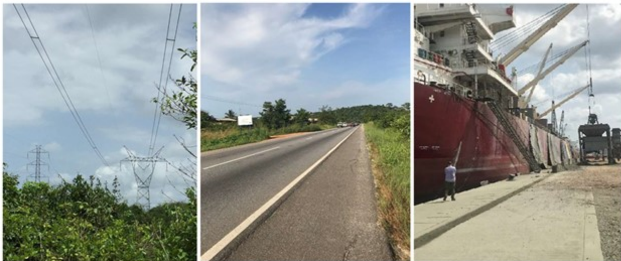
Figure 11: High voltage power transmission lines, bitumen highway and deep-sea Takoradi port close to project site.
