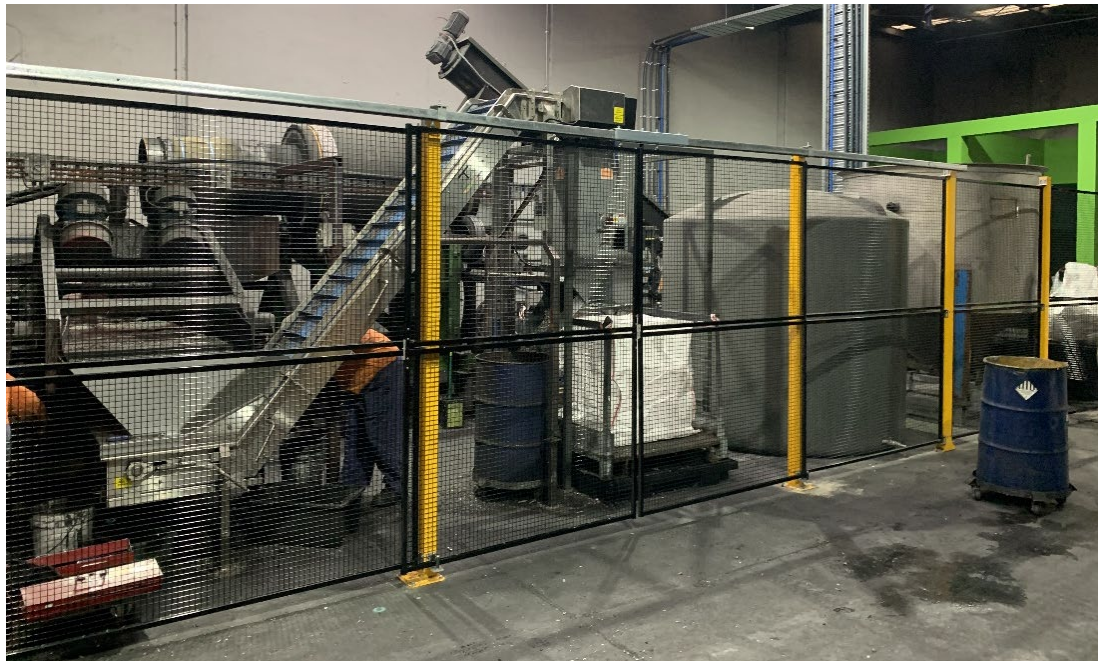
Berwick Road, Campbellfield Water Circuit Project – Wash Plant Upgrades
