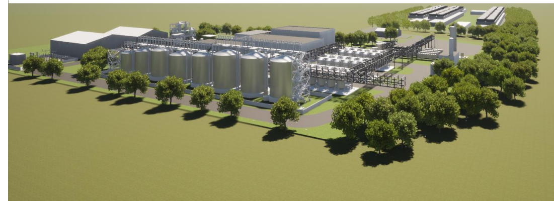
Top: construction of Lithium Extraction Optimisation Plant (LEOP) plant Bottom: Planned new commercial Phase One geothermal and LEP development.
