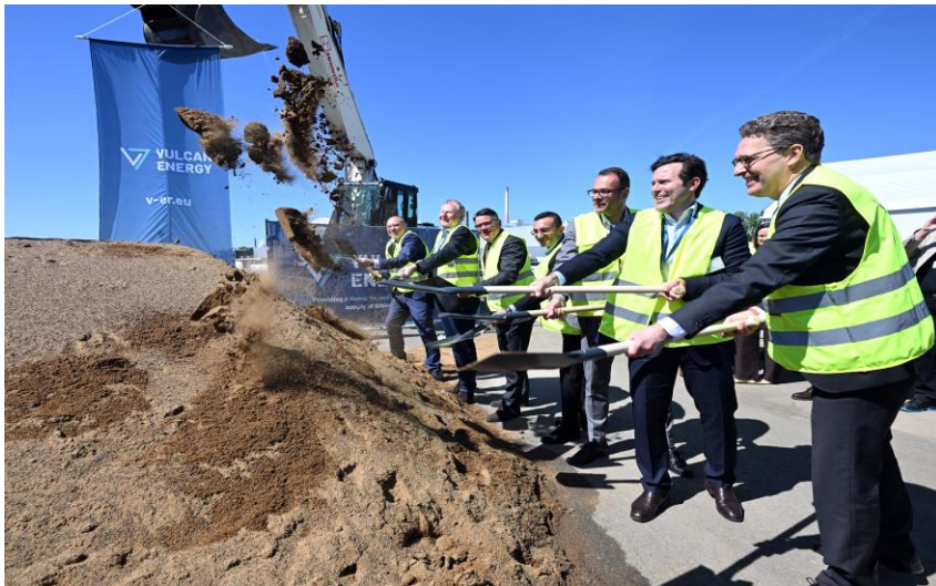
Groundbreaking at lithium chemical site in Frankfurt
