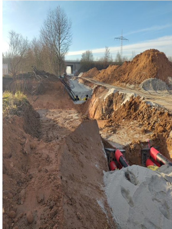
From left to right - relocation of the 110kV overhead power lines, underground power cables to replace overhead and drainage works at the integrated geothermal and lithium extraction site near Landau. Far right - concrete cellars for the new well pad at one of the new production well sites.
